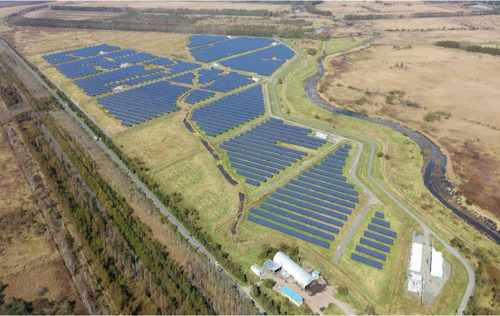
3. Overall view of Kushiro Toritoushi Wildland Solar Power Plant
