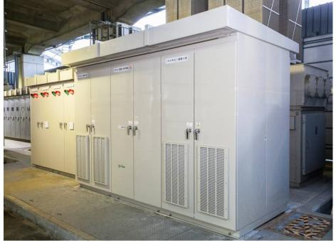
3. LIM25H-8 regenerative absorption lithium-ion battery
