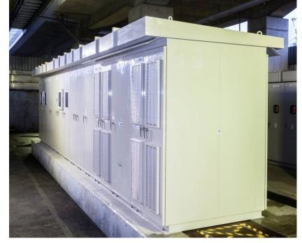
2. Emergency running storage batteries of the regenerative power storage system
