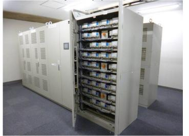
2. Anti-disaster power conditioners equipped with lithium-ion battery (organic thin film solar cells)
