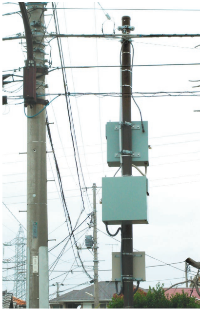
Fig. 1 Example of setting up power-supply system.
