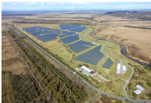
Overall view of Kushiro Toritoushi Wildland Photovoltaic Generation Plant
