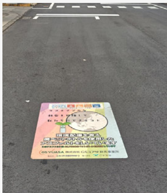
Environmentally considered road pavement on the premises (Gunma Plant)
