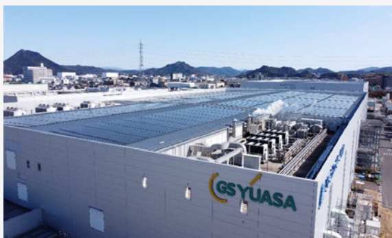
Solar power generation system
