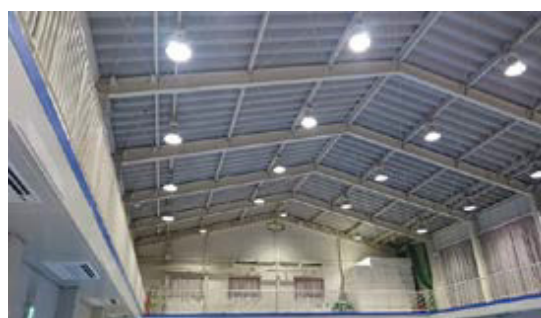
New LED lighting in the arena section of the gymnasium
