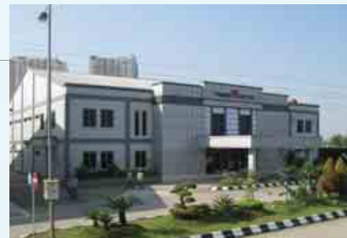
Front gate of head office
