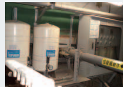
Facility for recycling cooling water 冷却水的循环设备
